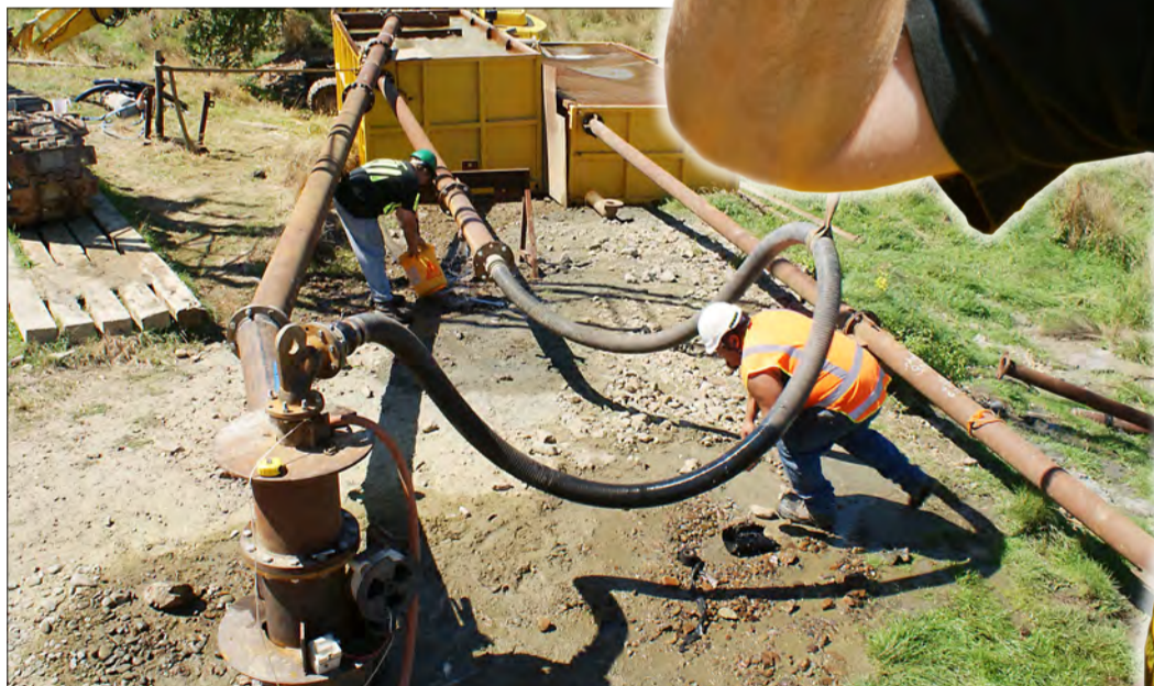
The new production bore near Ngarara Road. The bore is in the foreground left. In the distance are the two settling tanks
