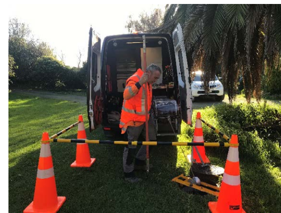
Stormwater pipe inspections with a CCTV camera to check for blockages, May 2019
