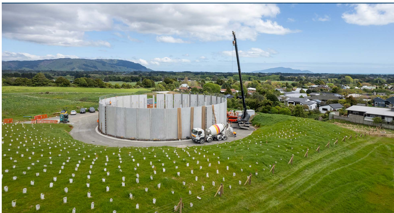
Ōtaki water reservoir construction
