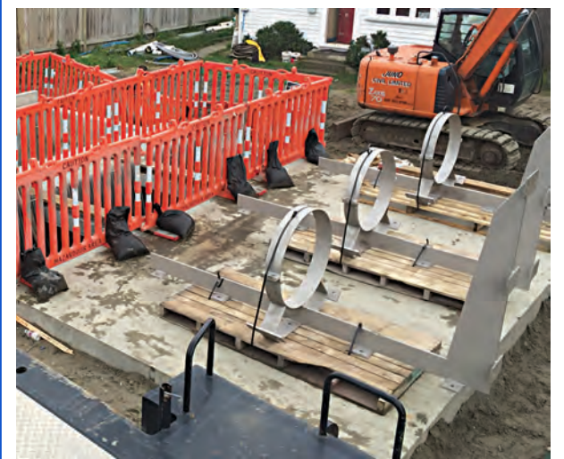
The new pump station under construction.
