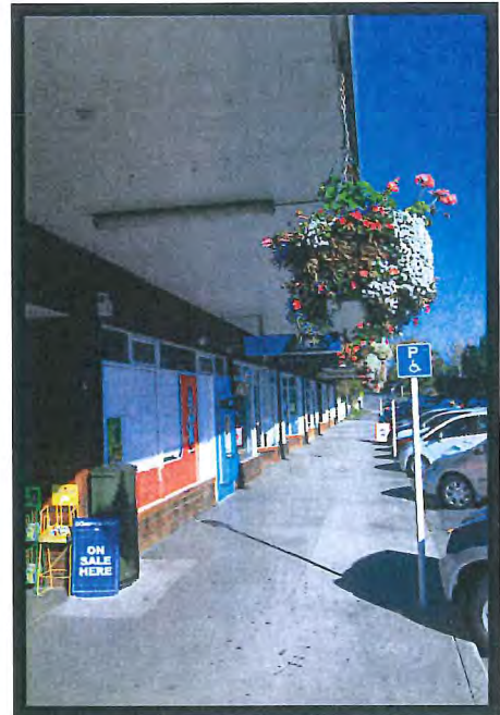
Active frontage and simple landscaping can delineate ownership and instil sense of place
