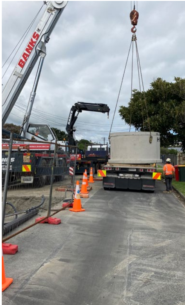
Installing a 2.5m diameter manhole at Ōtaki Beach
