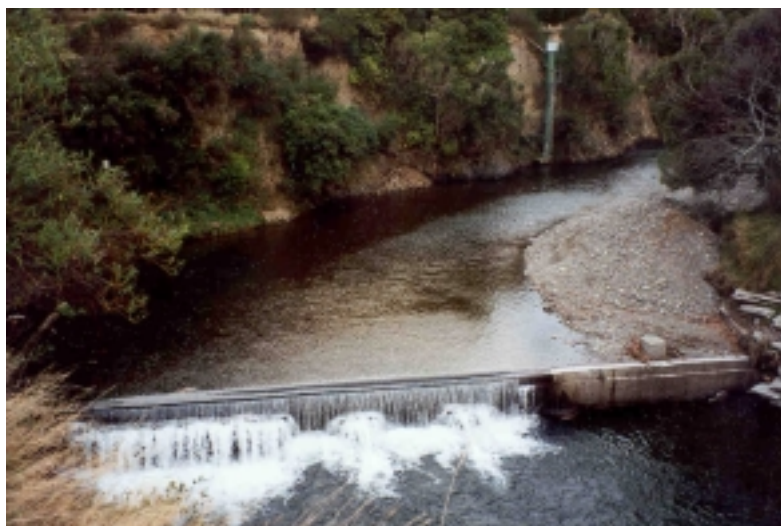
The Waikanae River intake. Flow is pumped from the river into the Waikanae Water Treatment Plant, to supply Waikanae, Paraparaumu and Raumati. In the background is the Waikanae River flow recording station.
