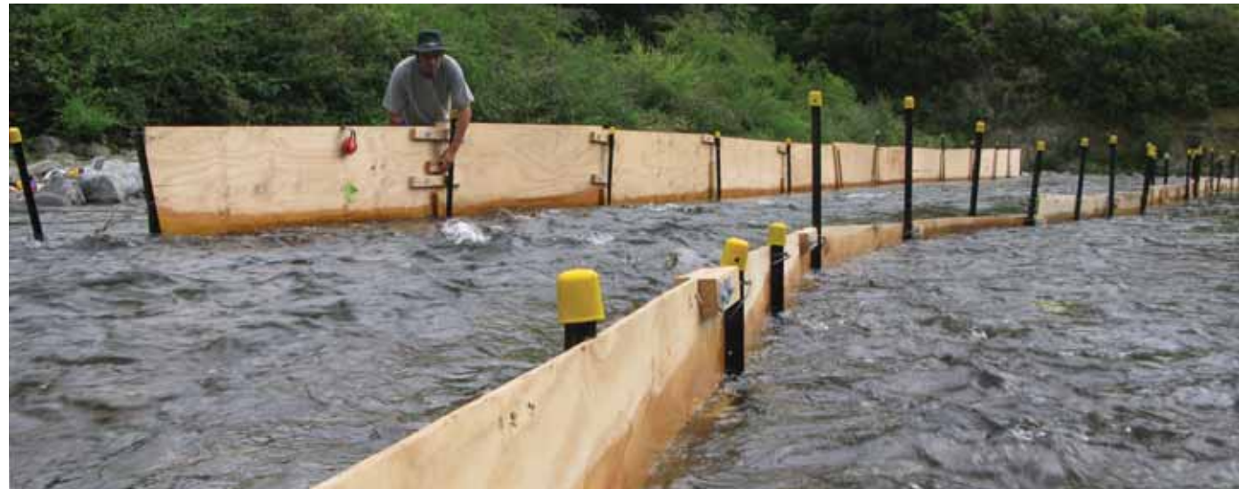
Dr Alastair Suren finishes the last of the river baffle installations.
