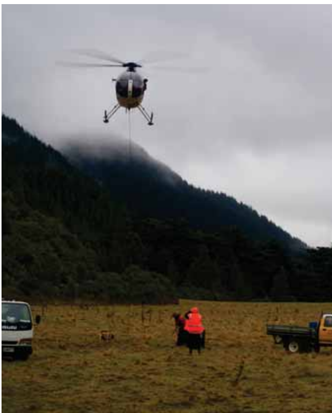
Helicopter moves drilling equipment for geotechnical testing
