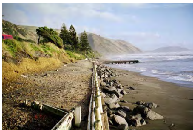
Fig 3.6: Rock and Timber Seawall at Raumati South
