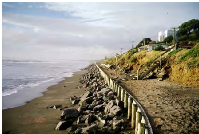
Fig 3.4: Rock and Timber Seawall Along The Parade
