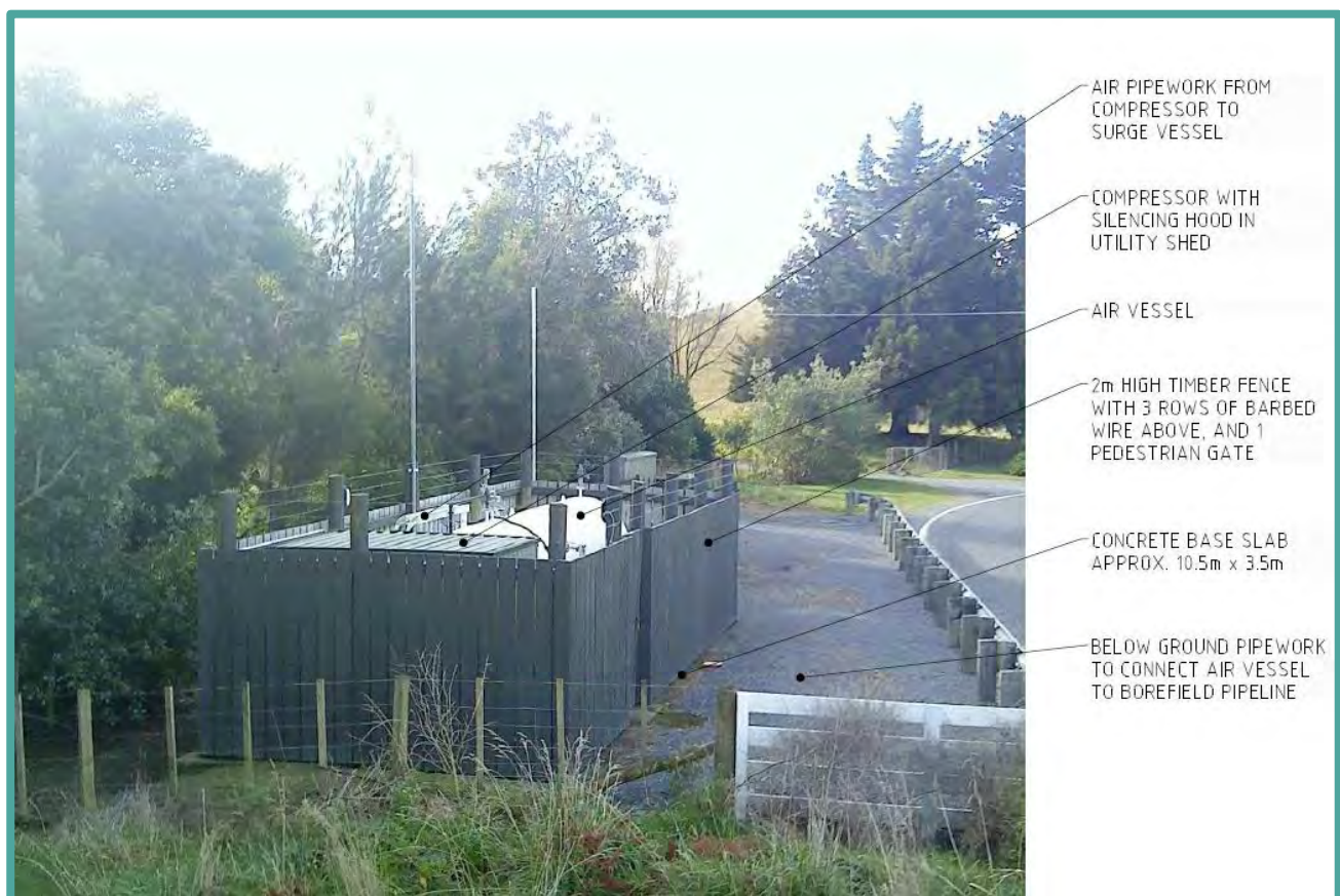
Figure 6 - Typical surge vessel arrangement
