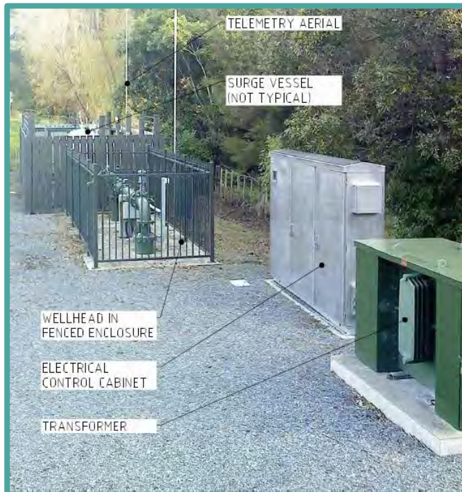
Figure 5 - Typical above ground wellhead arrangement
