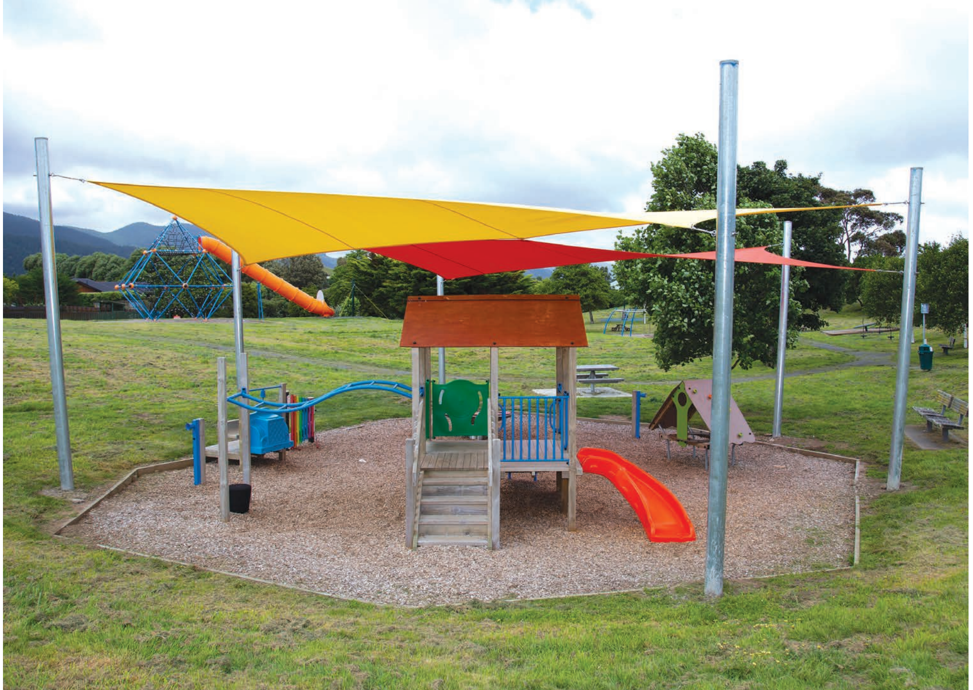
Mazengarb playground gets new shade sails installed.
