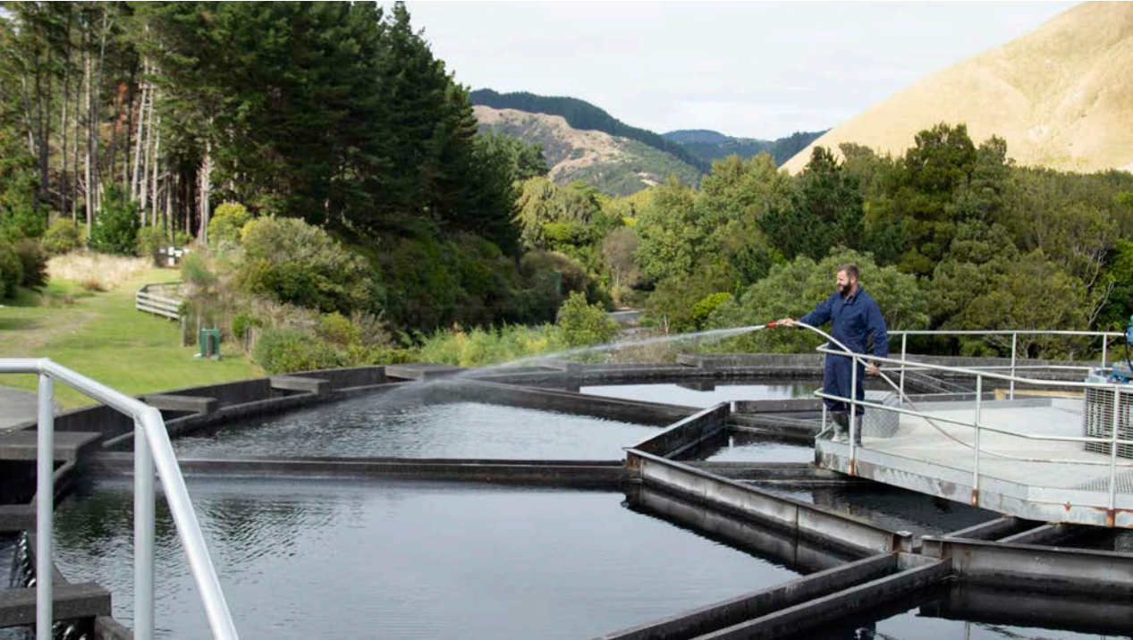
Waikanae Water Treatment Plant.
