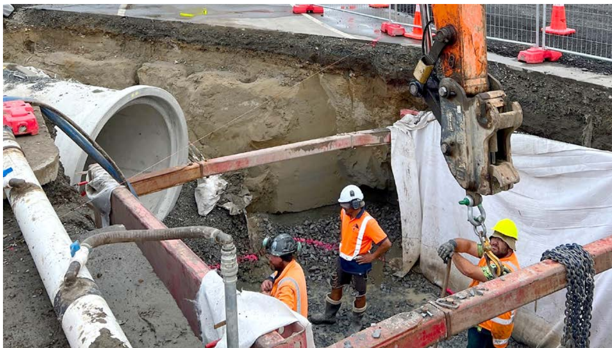
Amohia stormwater pipe installation.
