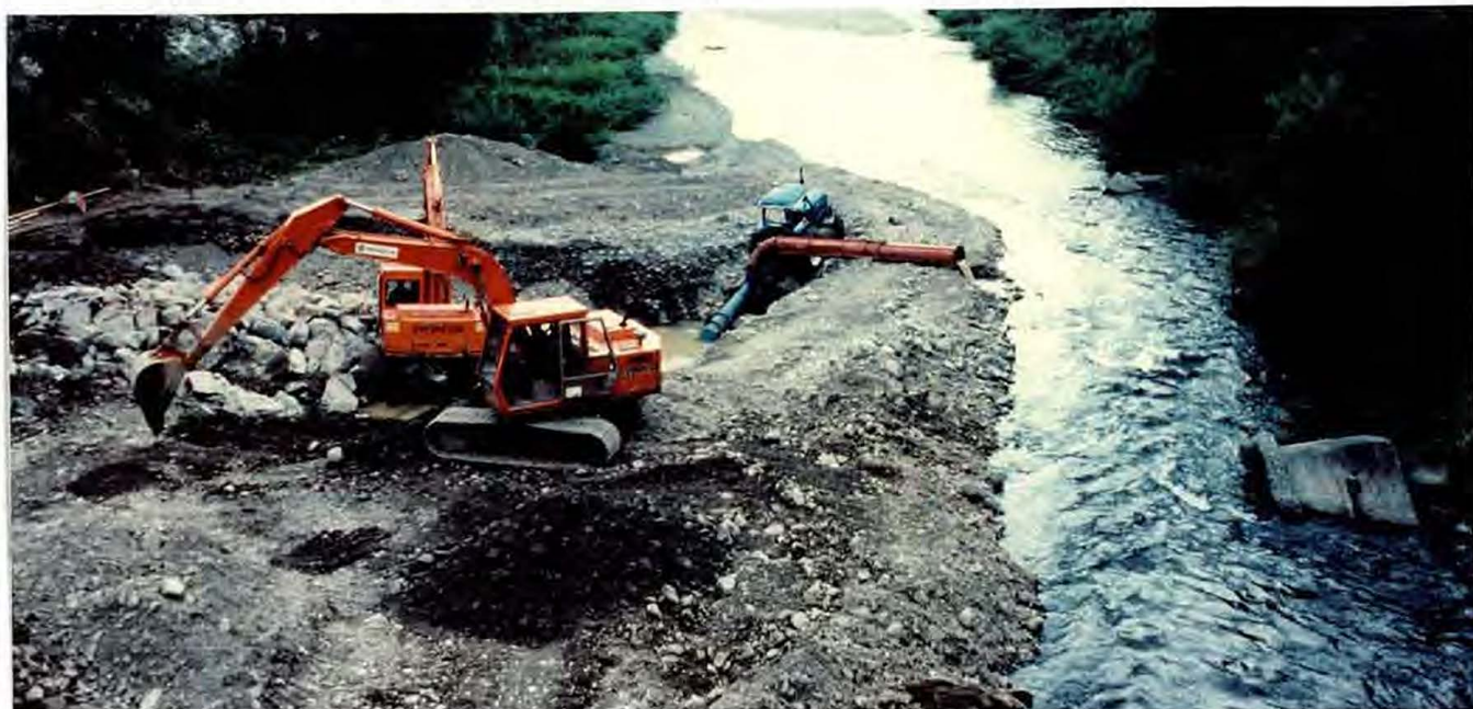
Figure 7. Ministry of Works construction of the Waikanae weir to control bed levels downstream of the state highway bridge. The rock weir replaced a concrete block weir that had been constructed and maintained by the catchment boards.
