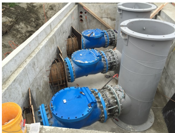
Ōtaki Beach pump station
