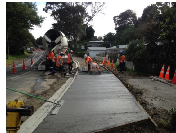
Poplar Avenue shared path under construction
