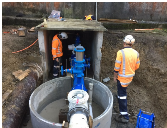
Auto shut-off valve installed at Kākāriki reservoir
