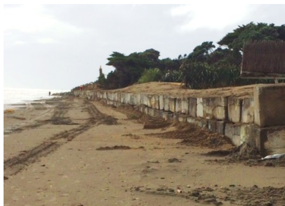
Wharemauku temporary block wall – built in three days following storm damage
