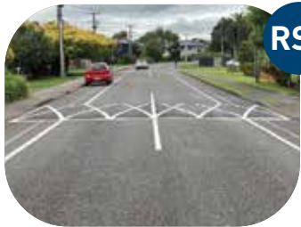
Construct Hump/ Platform
