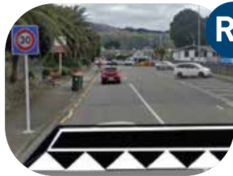
Raised Threshold Treatment
