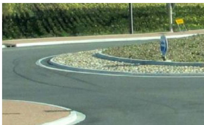
Photo 5 – Example of raised and textured roundabout apron
