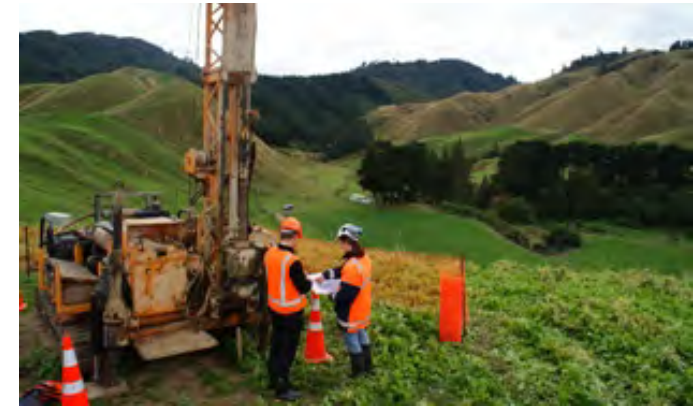
Drilling equipment for geotechnical testing
