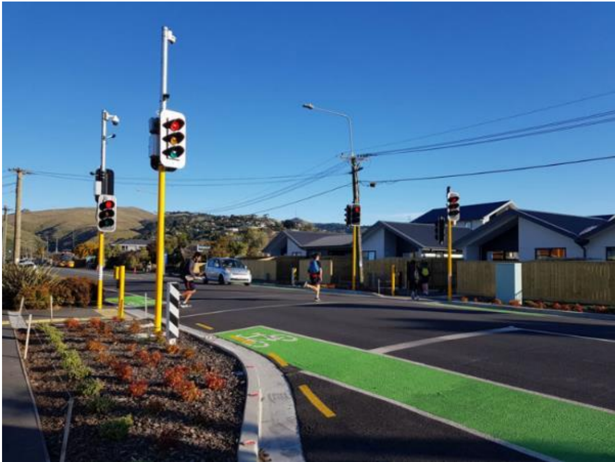
Image 9 Mid-block traffic signal controlled crossing example – Wilsons Road, Christchurch (Source Signalised crossings | Waka Kotahi NZ Transport Agency (nzta.govt.nz) )
