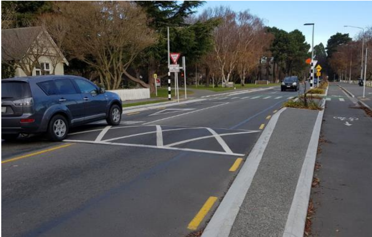
Image 13 Dual (un-raised) zebra crossing with vertical traffic calming example– Ilam Road, Christchurch (source Unsignalised crossings | Waka Kotahi NZ Transport Agency (nzta.govt.nz) )
