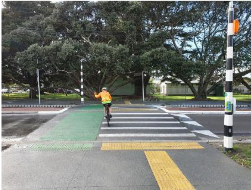
Image 6 –raised dual cycle/zebra crossing example - Carrington Road/Sutherland Road, Mount Albert, Auckland (source Unsignalised crossings | Waka Kotahi NZ Transport Agency (nzta.govt.nz) ).
