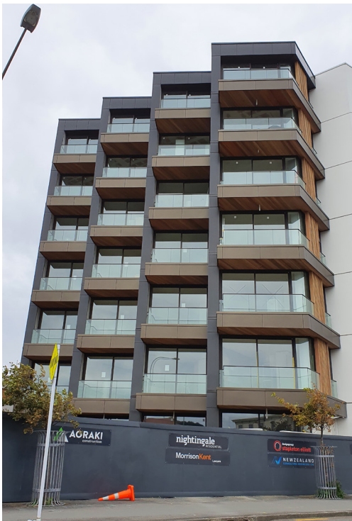
PHOTO 14 - STAGGERED BALCONIES MAXIMISE PRIVACY WHILE RETAINING OUTLOOK AND SUNLIGHT ACCESS (WELLINGTON)
