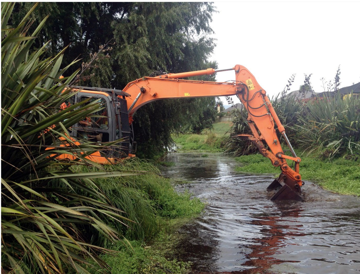
Digger clearing the Mazengarb Stream in Paraparaumu to minimise flood risk.
