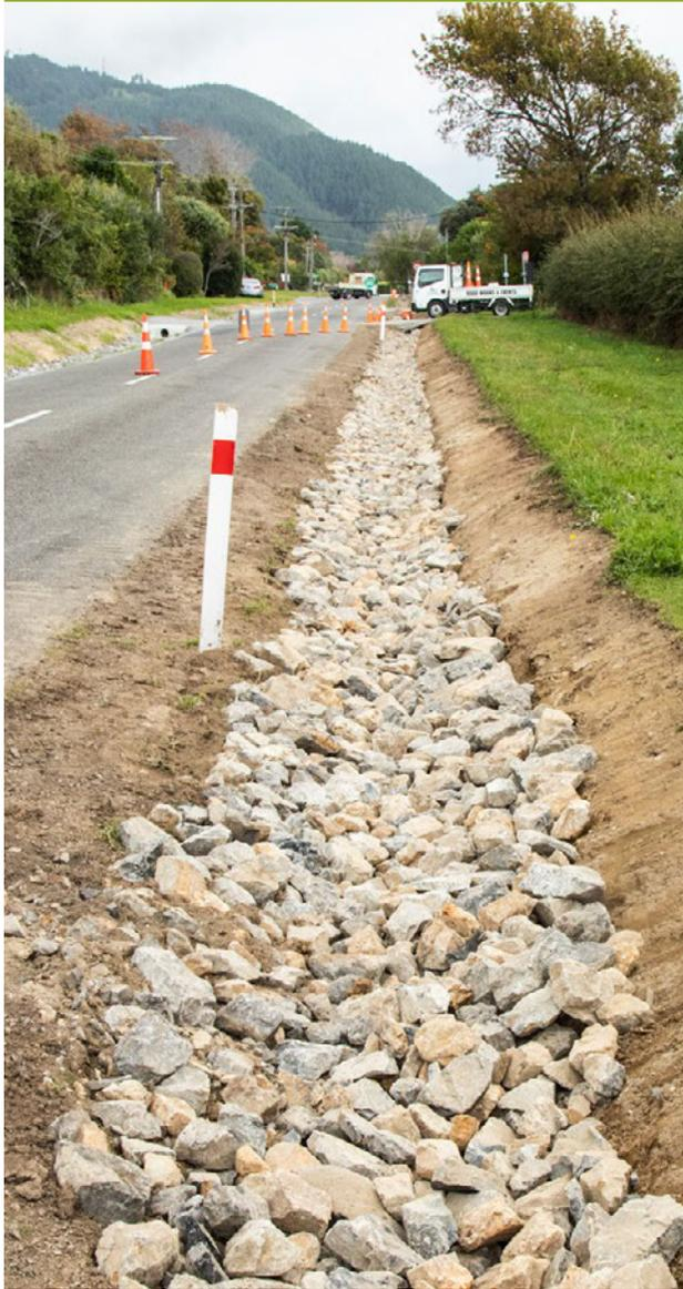
Run-off area works, Settlement Road, Te Horo. With increasing storms and heavy rainfall, our stormwater programme is a significant part of our response to climate change impacts.
