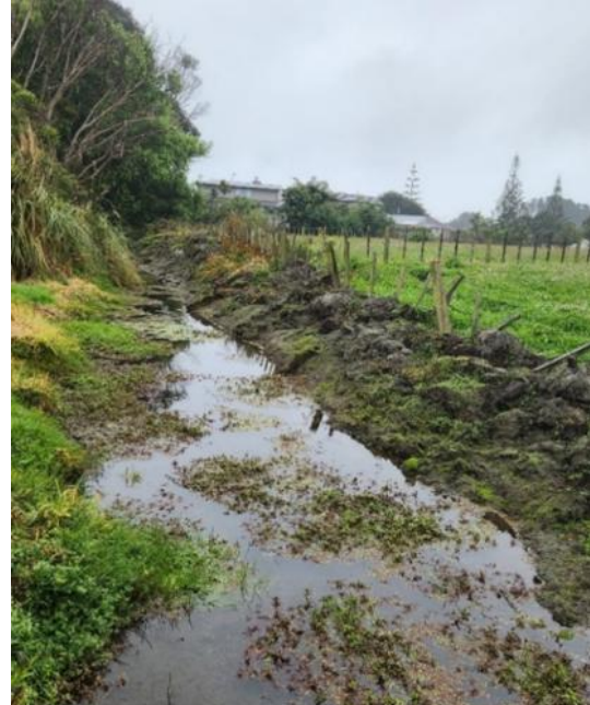
Photograph 4: Looking west along the watercourse from my site visit on 16 December 2024, showing a drop in water level within the stream correlating with a decrease in water level within the QEII wetland
