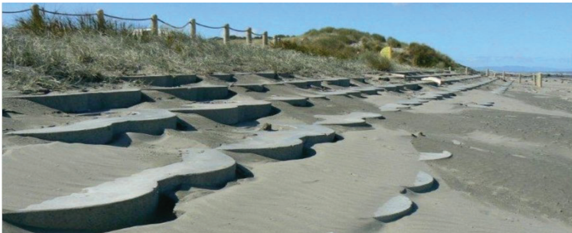
Stepped wall in Foxton saved the carpark and encouraged sand to return
