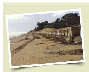
Following a one-in-30-year storm event in July 2016, a temporary block wall was installed within three days to protect the sewer from further damage.
