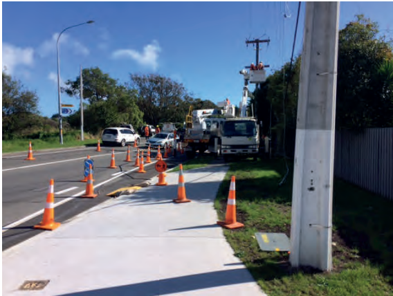
Undergrounding of overhead services on Te Moana Road before footpath widening can proceed
