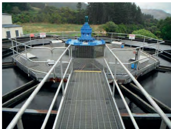
The clarifier at the Waikanae water treatment plant showing the central mixing area and surrounding settlement areas
