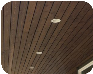
Use hardwood timber battens to tidy up the underside of existing awnings
