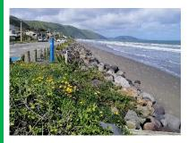
**2.** Enhance existing erosion protection structures (e.g. sea walls) Adding material to existing structures (e.g. sea walls) to increase resilience. This could include adding height to the top of the structure, as well as material to the toe to reduce toe scour and resulting failure.
