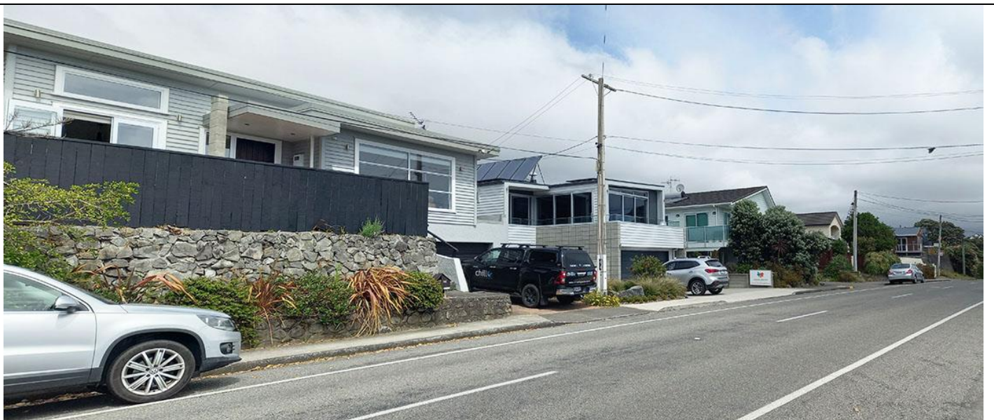
Photo 3. 2 Storey dwellings open to road frontage – 190, 192, 194, 196 Rosetta Road
