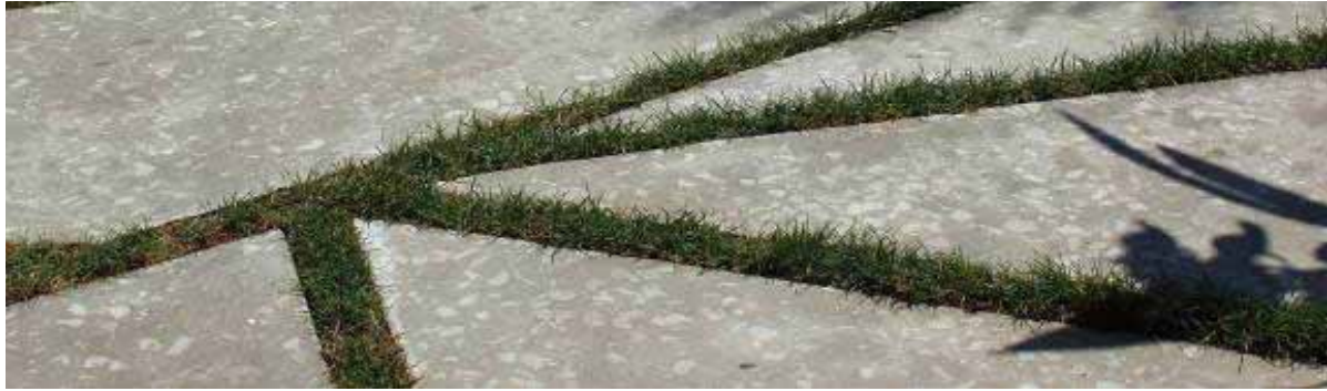
Figure 29: 'Friendly' concrete – relatively large gaps between pavers planted in grass or broadleaved groundcovers – reduces runoff. Photo: Robyn Simcock
