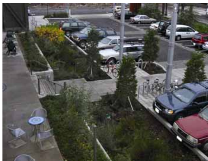
Figure 23: Planter boxes can treat stormwater from patios and roofs. Portland, Washington, USA. Photo: Marjorie van Roon
