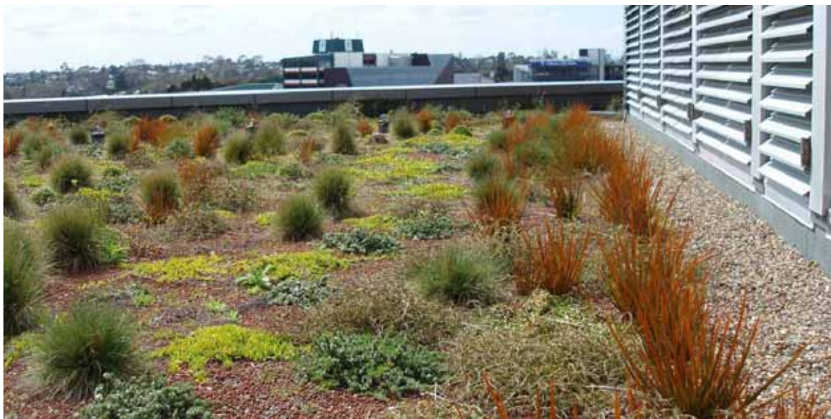
Figure 20: Waitakere Civic Centre (New Zealand) extensive green roof at about 16 months old. Extensive roofs are generally self-watering from rainfall. Photo: Robyn Simcock
