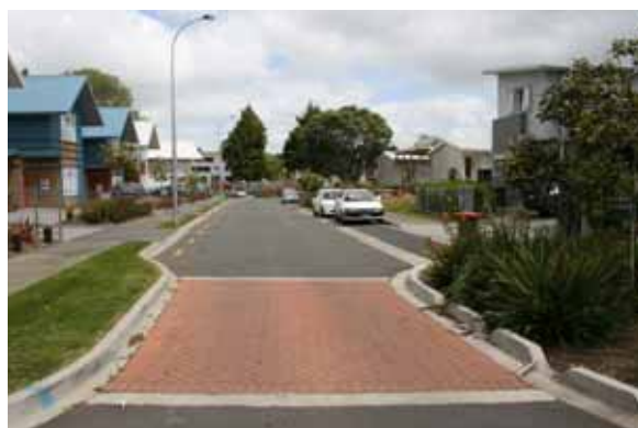
Figure 11: Narrow road, Talbot Park subdivision, Auckland, New Zealand. Raingarden on right treating road runoff and forming a traffic-calming feature. Photo: Maria Ignatieva
