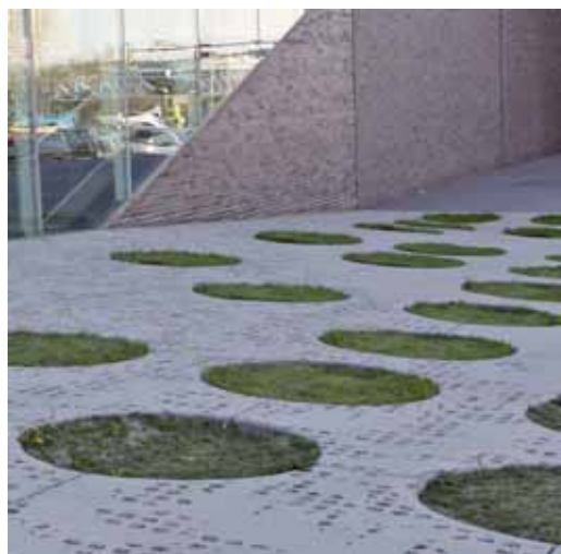
Figure 36: Mini-soakage areas (non-linear swales) with grass inset add interest to and reduce runoff from a large paved area outside an art gallery, Minneapolis, Minnesota, USA. Photo: Robyn Simcock
