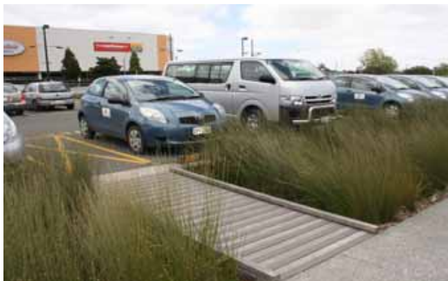
Figure 37: Bioretention strip planted mainly with oioi, rushes and other sedges. The wooden walkway covers an overflow structure. Waitakere City Centre car park, Auckland, New Zealand. Design: Meghan Wraight, Wraight & Associates. Photo: Maria Ignatieva
