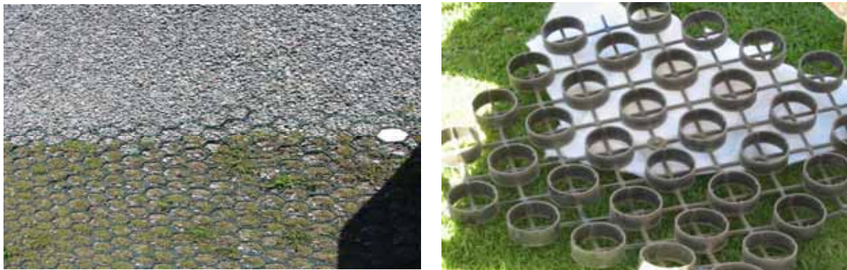
Figure 30 (a) and (b): Strong plastic grids increase bearing strength, reduce compaction of substrate, and allow plants to grow. Melbourne, Australia. Photos: Marjorie van Roon
