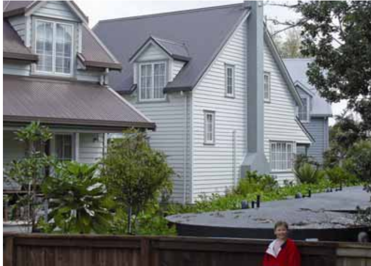
Figure 25: A series of half-buried rain tanks partly screened with native shrubs, Russell, Bay of Islands. Photo: Robyn Simcock
