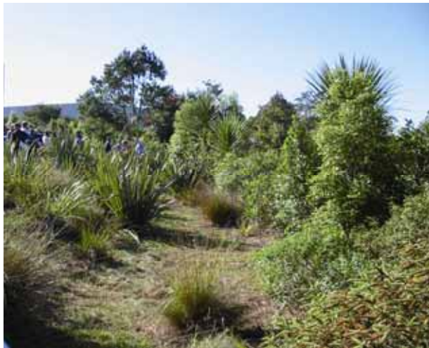
Figure 33: Vegetated swale behind the building previously tenanted by Waitakere City Council in Henderson. Photo: Marjorie van Roon
