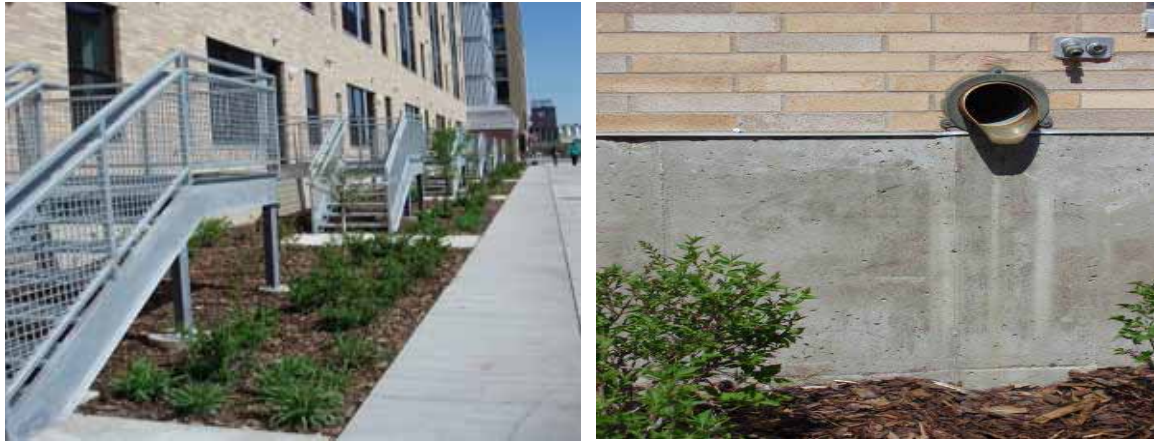
Figure 42 (a) and (b): Raingardens with minimal ponding depth in downtown Minneapolis, Minnesota, USA – right is the outlet to the downpipe – in this case a deep bark mulch replaces the more usual and longer lasting stones underneath the discharge point. Photo: Robyn Simcock
