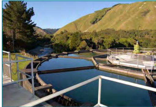
The Waikanae Water Treatment Plant
