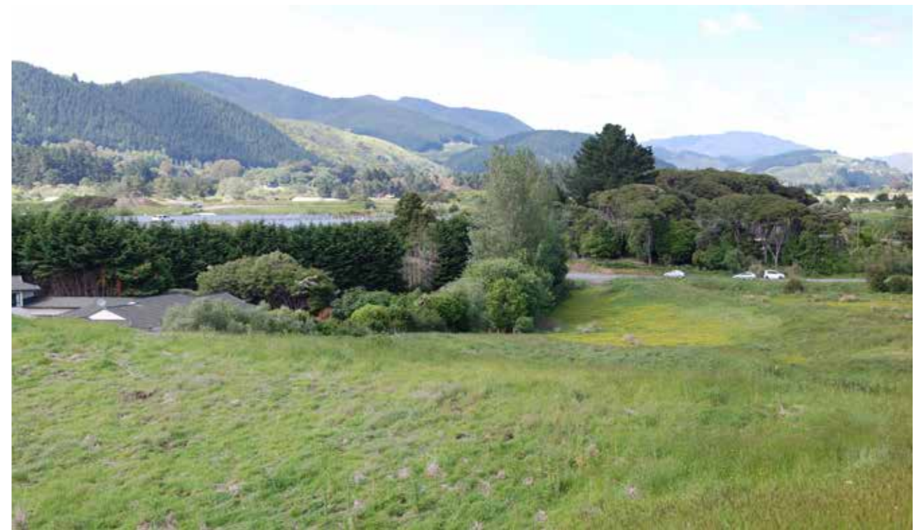
D Character - The character of the receiving environment is rural residential on the fringe of suburban development. The construction of the expressway has had a significant effect on the character of the receiving environment with changes to the topography, removal of vegetation and the installation of infrastructure.
