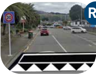
Raised Threshold Treatment
