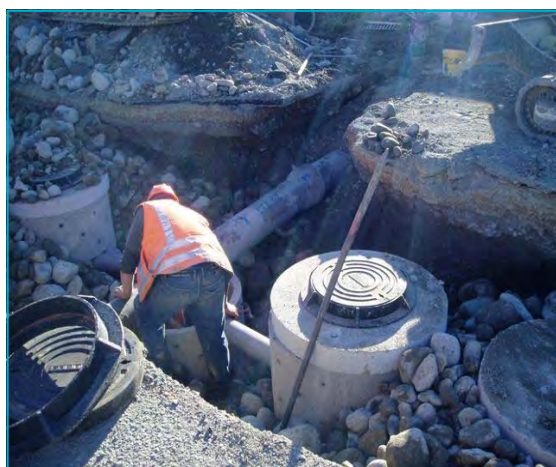
Installing stormwater pipes under a new road
