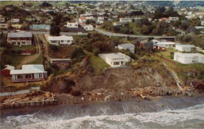
A. Coastal erosion behind failed structures on Rosetta Road following a significant storm in 1976.
