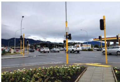
Intersection upgrade complete
