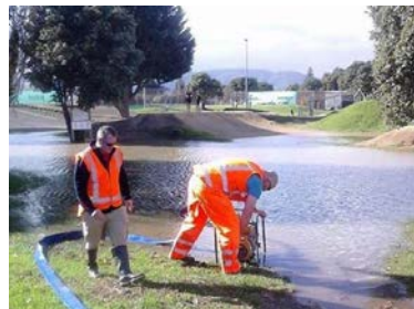
Pumping out floodwaters
