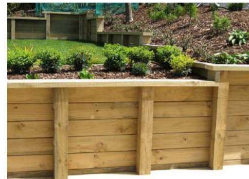
Timber Boundary Retaining Wall
