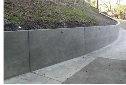
Concrete Boundary Retaining Wall
