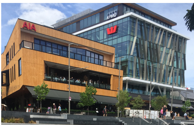
PHOTO 9 - BULK OF THE BUILDINGS BROKEN DOWN BY LAYERS (BOTTOM, MIDDLE, TOP), CHRISTCHURCH.
