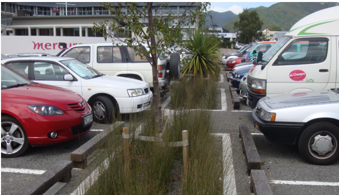
PHOTO 3 - LANDSCAPE TREATMENT AND RAIN GARDENS AS PART OF PARKING LOT
