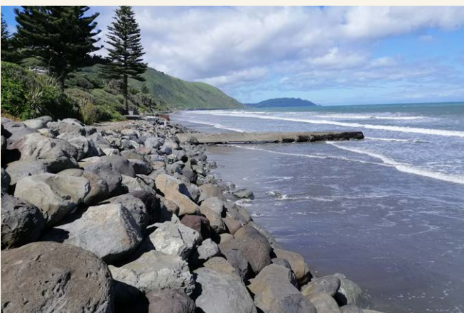
C. Paekākāriki seawall at Beach Road.
