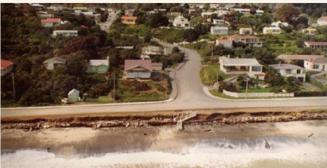
B. Structure failure and coastal erosion following September 1976 storm.
