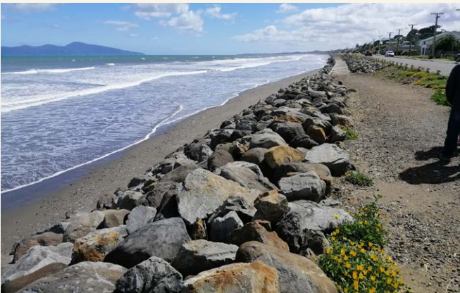
A. Rock revetment structure along The Parade.
