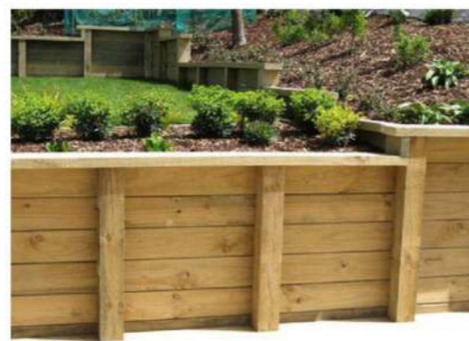
Timber Boundary Retaining Wall
