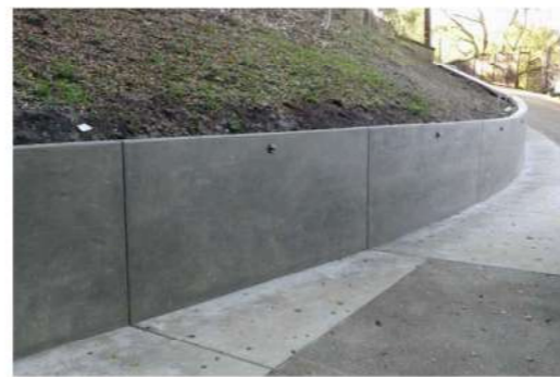
Concrete Boundary Retaining Wall
