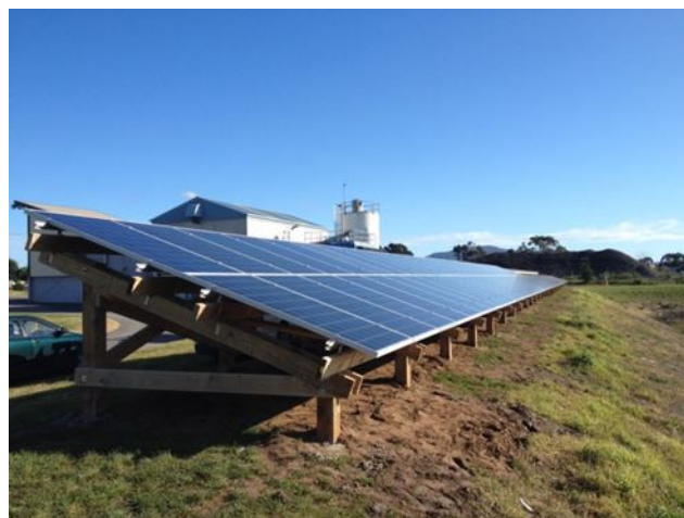
Pilot solar array at the Paraparaumu wastewater treatment plant providing cheaper electricity.
