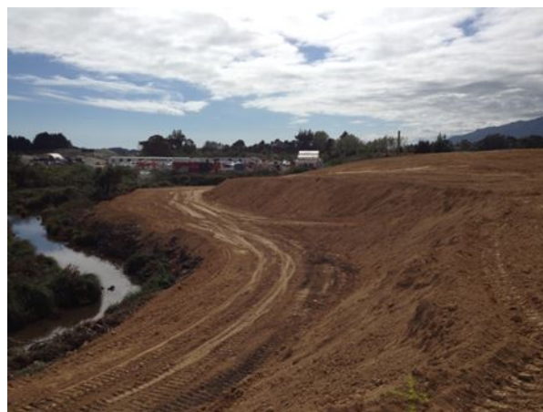
Capping underway at Otaihanga landfill
