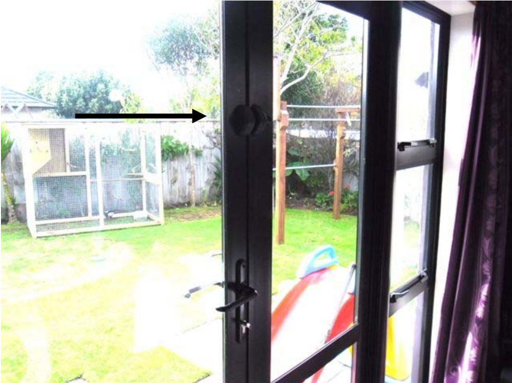
Opening door - release bolt at 1.5 metres above floor
