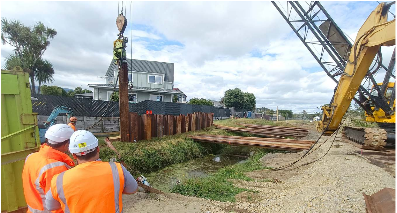
Contractor installing sheet piles ahead of building foundations and walls for the pump that will be installed as part of the Kenakena stormwater upgrade.
