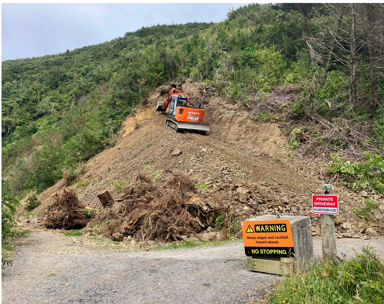
Earthworks started in February to clear the two slips at Blue Bluff on Ōtaki Gorge Road.
