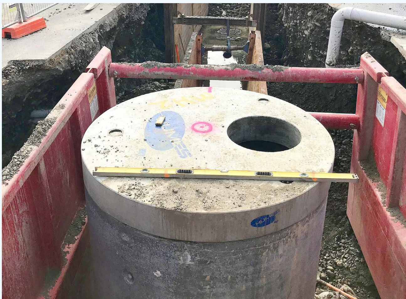
Installation of a manhole on Riverbank Road, Ōtaki.
