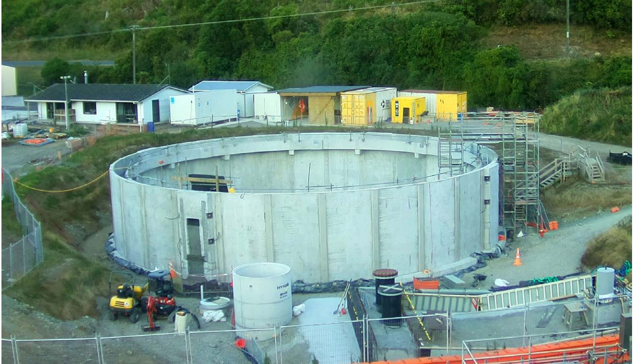
The new clarifier, a large tank which helps remove tiny particles from the river water, being built at Waikanae Water Treatment Plant.
