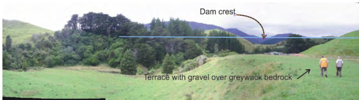
Figure 4-3: Kapakapanui Lower Dam Site Looking Downstream
