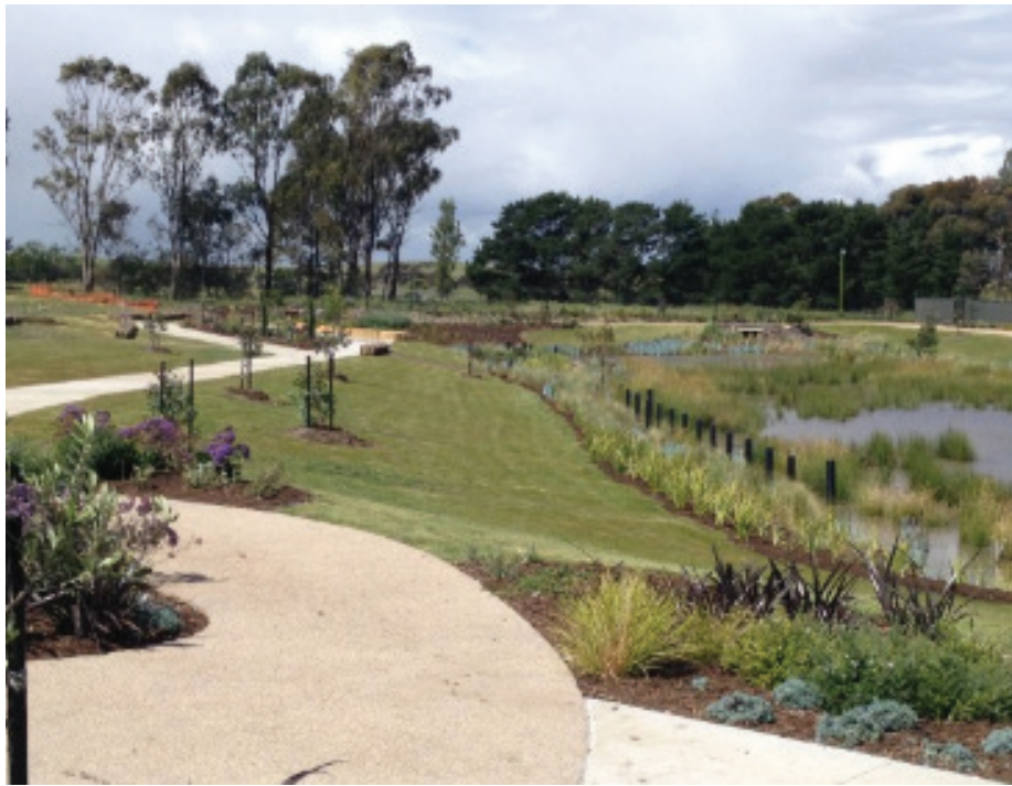
Stormwater reserve example
