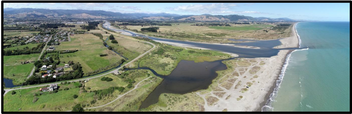
Figure 10: Aerial photo of the Ōtaki River mouth, 2020. (Source: Greater Wellington Regional Council) 50
