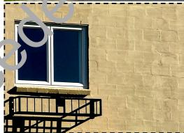
ABOVE: AN ENLARGED PORTION OF A POORLY FIN-ISHED DWELLING, WITH A PLASTER FINISH FAILING TO PROVIDE EITHER AN EVEN OR EFFECTIVE COAT-ING. THE CONCRETE BLOCK WORK IS CLEARLY VISI-BLE THROUGH THE FINISH, GIVING THE NEW DWELL-ING AN ALREADY BADLY AGED APPEARANCE.
