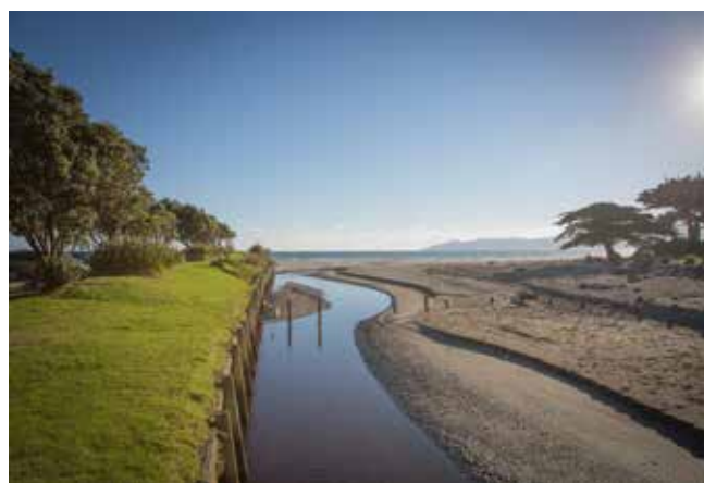
Effective stormwater management contributes to healthy waterways.
