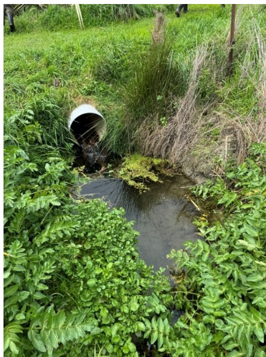
Photo A4.2. Downstream end of culvert, containing harakeke woven rope as a fish passage remediation tool.
