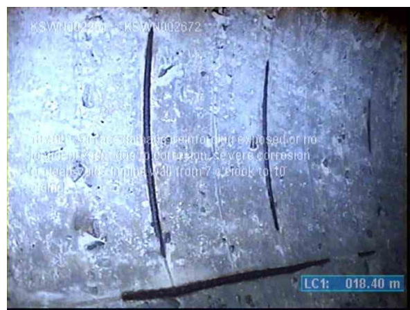
KSWP004512_0244a32f-c0b6-44dc-be00-d1b417667dd6_20220711_125619_066.jpg, 00:02:44, 18.40m Surface damage, reinforcing exposed or no longer present due to corrosion, severe corrosion or deep voids in pipe wall from 7 o'clock to 10 o'clock
