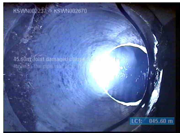
KSWP003713_bdd97187-9c4c-4e12-97c5-650296e93888_20220811_132048_371.jpg, 00:04:25, 45.60m (2.60m) Joint damaged/chipped, large, clearly through the pipe wall from 12 o'clock to 12 o'clock
