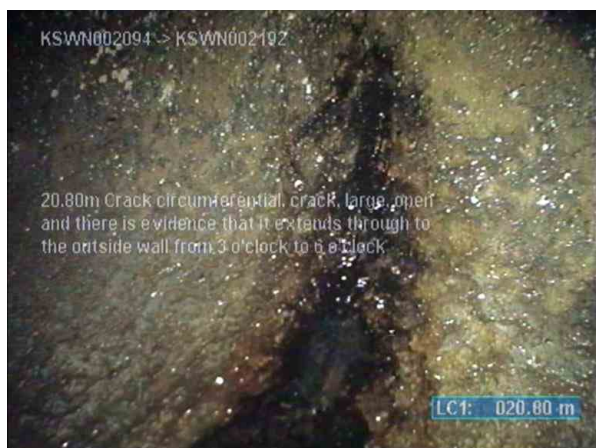
KSWP003817_db4cbf4f-896b-4697-8544-55b7a58b3b42_2020812_113238_708.jpg, 00:04:32, 20.80m (35.20m) Crack circumferential, crack, large, open and there is evidence that it extends through to the outside wall from 3 o'clock to 6 o'clock
