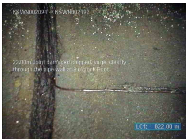
KSWP003817_bf9a678e-ebf6-4e9e-a17c-8ff011637ce3_20220812_113348_222.jpg, 00:05:24, 22.00m (34.00m) Joint damaged/chipped, large, clearly through the pipe wall at 9 o'clock / Root
