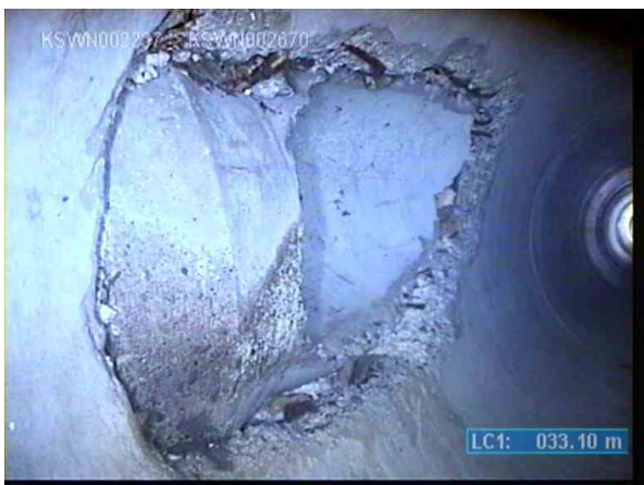
KSWP003713_ab94fea7-9b65-4da0-ae52-e7a3c67fc7da_2020811_131941_203.jpg, 00:03:14, 32.80m (15.40m) The lateral is open at 9 o'clock / Ok
