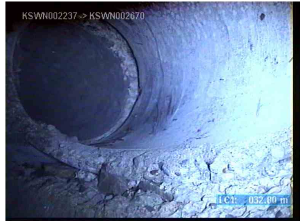
KSWP003713_ba39b8cc-c631-4d6d-bf67-e948ee438793_2020811_131924_634.jpg, 00:03:14, 32.80m (15.40m) The lateral is open at 9 o'clock / Ok
