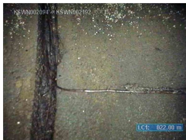
KSWP003817_da90fc7a-621a-40ac-8dd4-68883b6b4d57_20220812_113358_896.jpg, 00:05:30, 22.00m (34.00m) Fine roots, roots restrict flow by 10% or less of full flow at 9 o'clock
