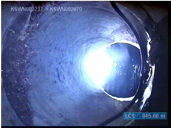
KSWP003713_4a77d837-2bba-4c40-a44b-a017512c4149_20220811_132102_186.jpg, 00:04:31, 45.60m (2.60m) Gap separation width 20mm
