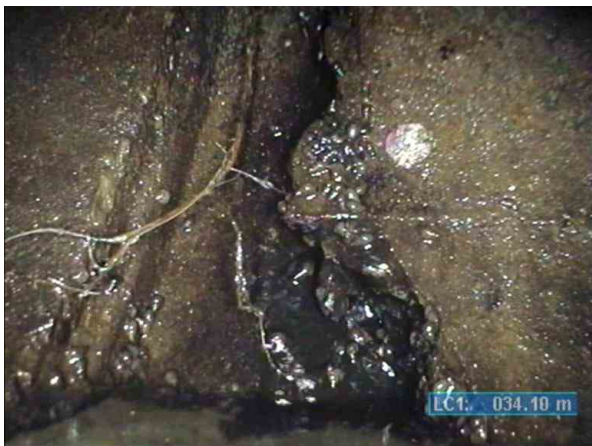
KSWP003817_700bbb4a-d05f-4d20-bcb1-caed32b5e03b_20220812_113613_212.jpg, 00:07:24, 34.10m (21.90m) Joint damaged/chipped, large, clearly through the pipe wall from 3 o'clock to 9 o'clock / Infiltration and broken
