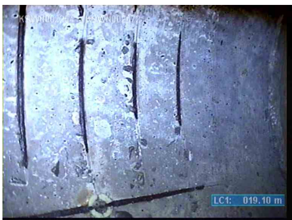
KSWP004512_060d03ac-41e2-4c53-bf61-835357fe24d4_20220711_125640_322.jpg, 00:03:03, 19.10m Surface damage, reinforcing exposed or no longer present due to corrosion, severe corrosion or deep voids in pipe wall from 7 o'clock to 10 o'clock
