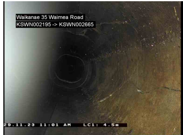
42_KSWP003751_200.jpg, 00:03:25, 4.50m (10.90m) Cracks multiple, medium, crack open but there is no evidence that the crack extends to the outside wall from 10 o'clock to 3 o'clock
