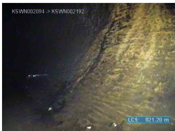
KSWP003817_0914ca62-fff3-4eec-9a37-9975186a6ff3_20220812_113311_329.jpg, 00:04:55, 21.20m (34.80m) Encrustation deposits, clear diameter is reduced by less than 10% from 3 o'clock to 6 o'clock
