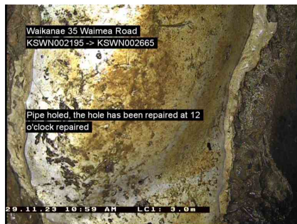
42_KSWP003751_196.jpg, 00:02:26, 3.00m (12.40m) Pipe holed, the hole has been repaired at 12 o'clock / repaired
