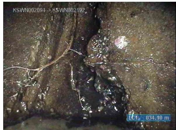
KSWP003817_adfc3087-874e-45aa-86b4-190dc5edbc04_20220812_113624_055.jpg, 00:07:30, 34.10m (21.90m) Infiltration, running (visibly moving) flow from 3 o'clock to 6 o'clock
