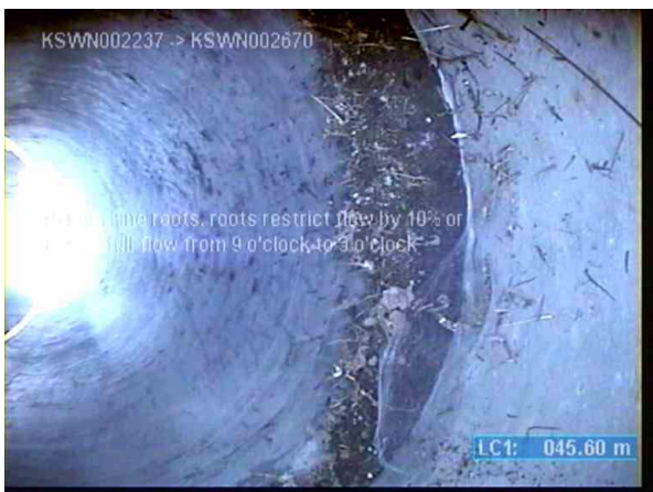
KSWP003713_90419e6e-c99a-4298-a253-86fee32ccced_20220811_132134_875.jpg, 00:04:52, 45.60m (2.60m) Fine roots, roots restrict flow by 10% or less of full flow from 9 o'clock to 3 o'clock
