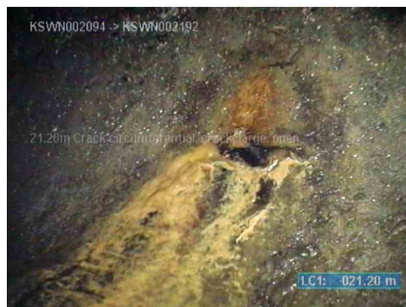
KSWP003817_17864e24-11e9-4cd5-acf6-a256721788ba_20220812_113319_750.jpg, 00:05:04, 21.20m (34.80m) Crack circumferential, crack, large, open and there is evidence that it extends through to the outside wall from 3 o'clock to 6 o'clock
