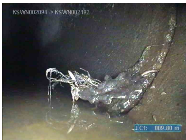
KSWP003817_c21fe9cd-398c-42ed-b7fb-1d5d78366c5d_2020812_113017_759.jpg, 00:02:25, 9.80m (46.20m) Fine roots, roots restrict flow by 10% or less of full flow from 4 o'clock to 6 o'clock
