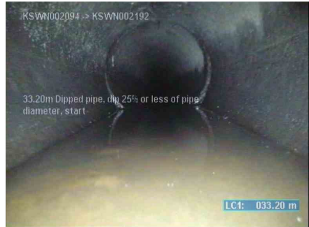
KSWP003817_c346b211-c8d1-4778-881d-df197c90eed6_20220812_113525_551.jpg, 00:06:53, 33.20m (22.80m) Dipped pipe, dip 25% or less of pipe diameter, start
