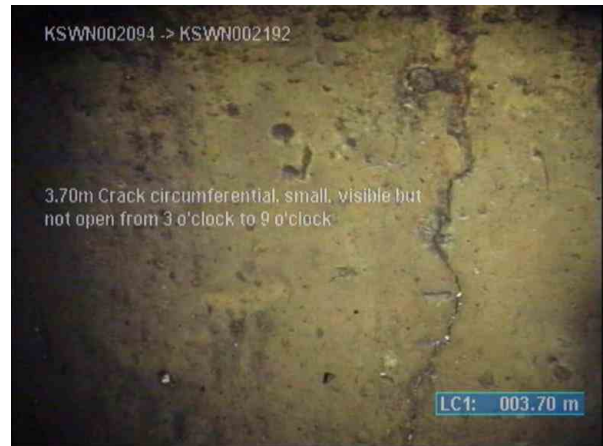
KSWP003817_06475611-4031-46c4-9258-8a08b54254d5_20220812_112909_255.jpg, 00:01:29, 3.70m (52.30m) Crack circumferential, small, visible but not open from 3 o'clock to 9 o'clock
