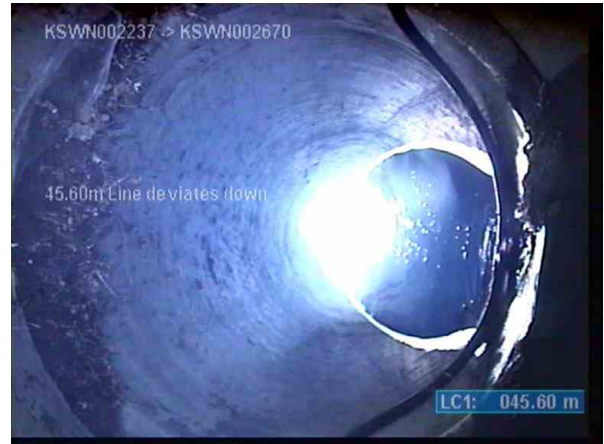
KSWP003713_71c9edd4-90be-4488-97db-24646cada9ca_20220811_132110_921.jpg, 00:04:37, 45.60m (2.60m) Line deviates down
