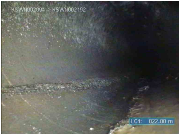
KSWP003817_af5911e6-1802-49a9-9655-90a61d5d830e_20220812_113403_886.jpg, 00:05:30, 22.00m (34.00m) Fine roots, roots restrict flow by 10% or less of full flow at 9 o'clock
