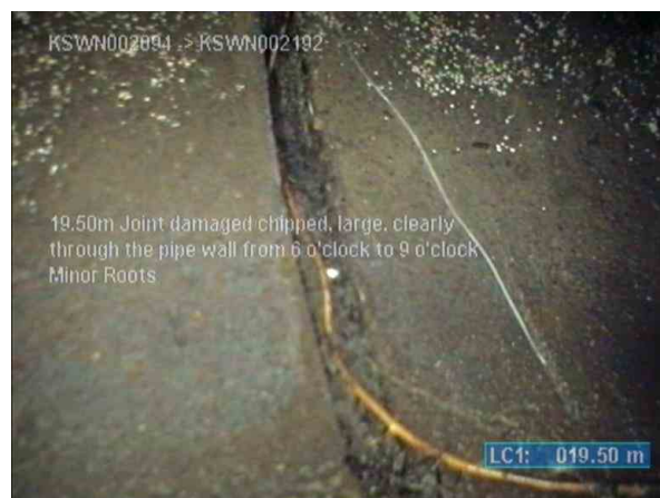
KSWP003817_36c32fb4-a4dc-41d3-aa9c-aab22b83395a_2020812_113157_910.jpg, 00:03:54, 19.50m (36.50m) Joint damaged/chipped, large, clearly through the pipe wall from 6 o'clock to 9 o'clock / Minor Roots
