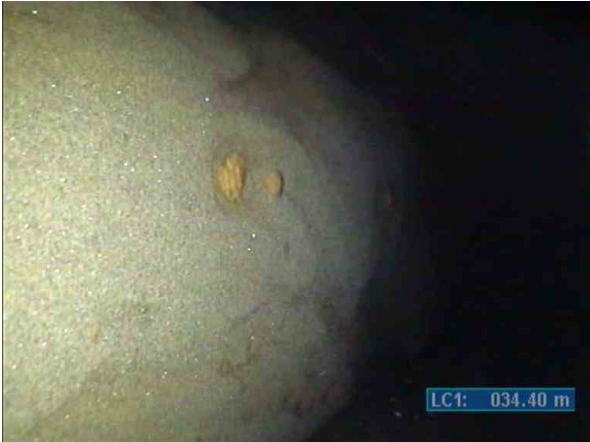
KSWP003817_87ccedcd-31e1-4b81-b037-d14fae2386ca_20220812_113645_304.jpg, 00:07:47, 34.40m (21.60m) Debris silt, small, clear diameter reduced by less than 10%, start
