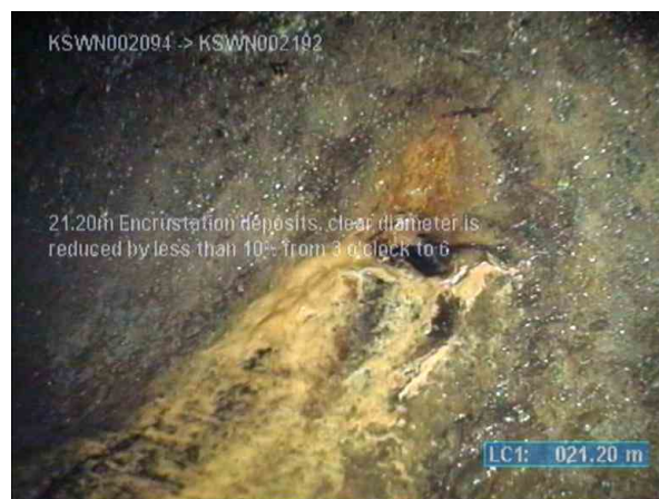
KSWP003817_c9bedc18-acc9-4587-be8a-7ff7d5d63b6e_2020812_113306_569.jpg, 00:04:55, 21.20m (34.80m) Encrustation deposits, clear diameter is reduced by less than 10% from 3 o'clock to 6 o'clock
