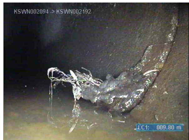
KSWP003817_35b78b62-6938-4352-9f91-7300c8ca4902_20220812_113006_929.jpg, 00:02:18, 9.80m (46.20m) Joint damaged/chipped, large, clearly through the pipe wall from 4 o'clock to 6 o'clock / Roots
