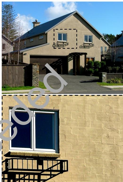
**ABOVE:** AN ENLARGED PORTION OF A POORLY FINISHED DWELLING, WITH A PLASTER FINISH FAILING TO PROVIDE EITHER AN EVEN OR EFFECTIVE COATING. THE CONCRETE BLOCK WORK IS CLEARLY VISIBLE THROUGH THE FINISH, GIVING THE NEW DWELLING AN ALREADY BADLY AGED APPEARANCE.
